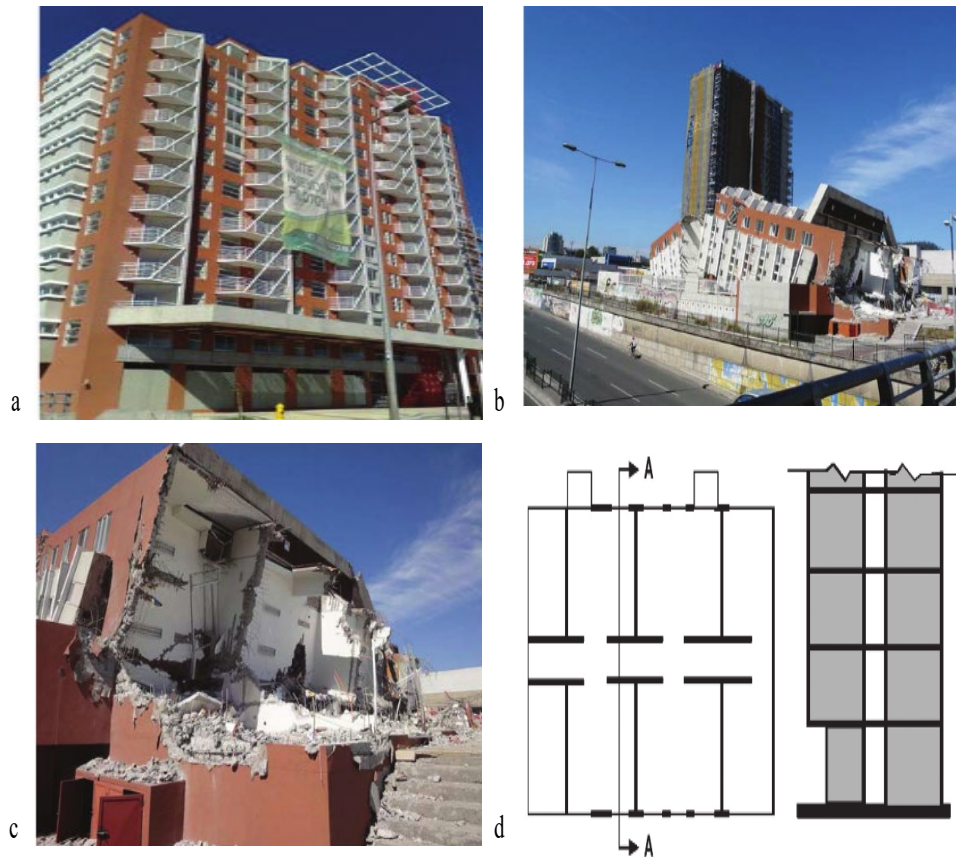
FIGURE 2.1: Alto Rio Condominium building in Concepcion; (a) building prior to earthquake, (b) building post-earthquake, (c) failure of shear wall, and (d) approximate plan of building [7]
