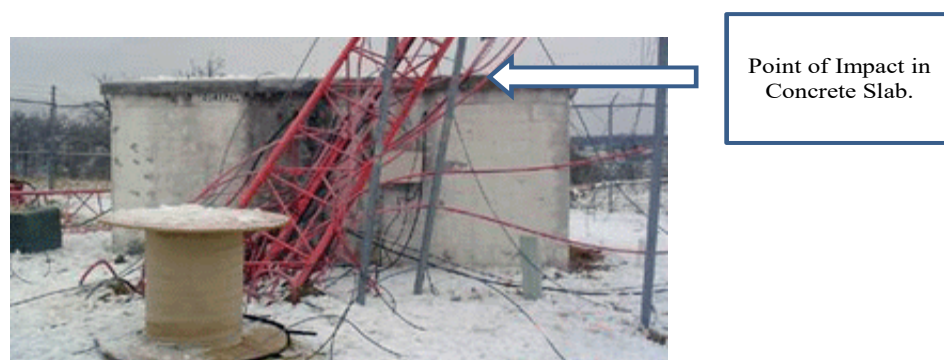
FIGURE 2.1: Collapse of tower on slab.
