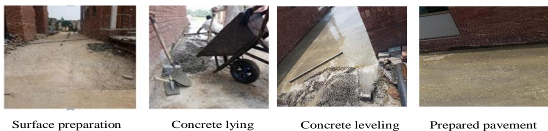
FIGURE 5.2: Wheat straw fiber reinforced concrete pavement [114]
