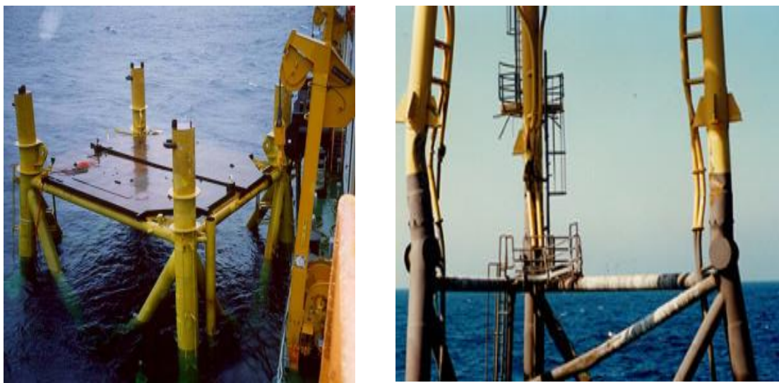
FIGURE 2.2: Offshore jacket platform, a) Studied structure [14], and b) Damaged offshore jacket structure due to impact load
