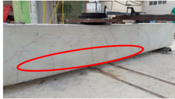
Cracks in Beams
