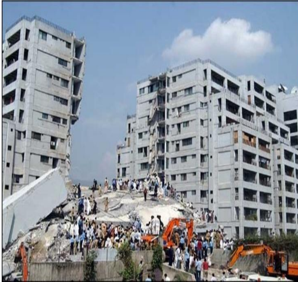
FIGURE 2.3: Collapse of Margalla tower during earthquake 2005
