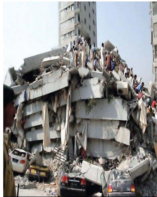
b) Structural collapse
