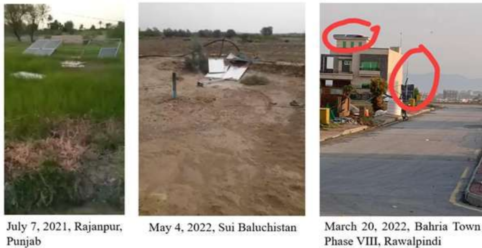
FIGURE 1.16: Damages caused by Wind at Different Locations
