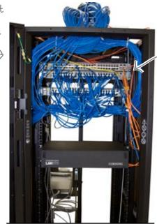
The horizontal cable management tray keeps cable from falling in front of other things in the rack.
