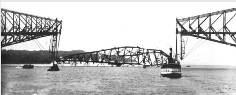
Photo 1.4 — The Quebec Bridge (1916 collapse). The collapse of the centre span of the Quebec Bridge (St. Lawrence design), photographed at the instant it hit the water on September 11, 1916.
