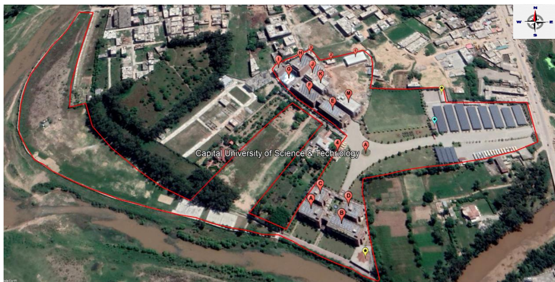
FIGURE 4.1: Aerial view of CUST show Soan River
