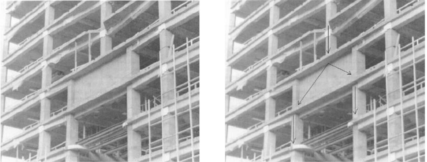
Figure 2.3. Single Span Deep Beam (MacGregor & Wight, 2005)
