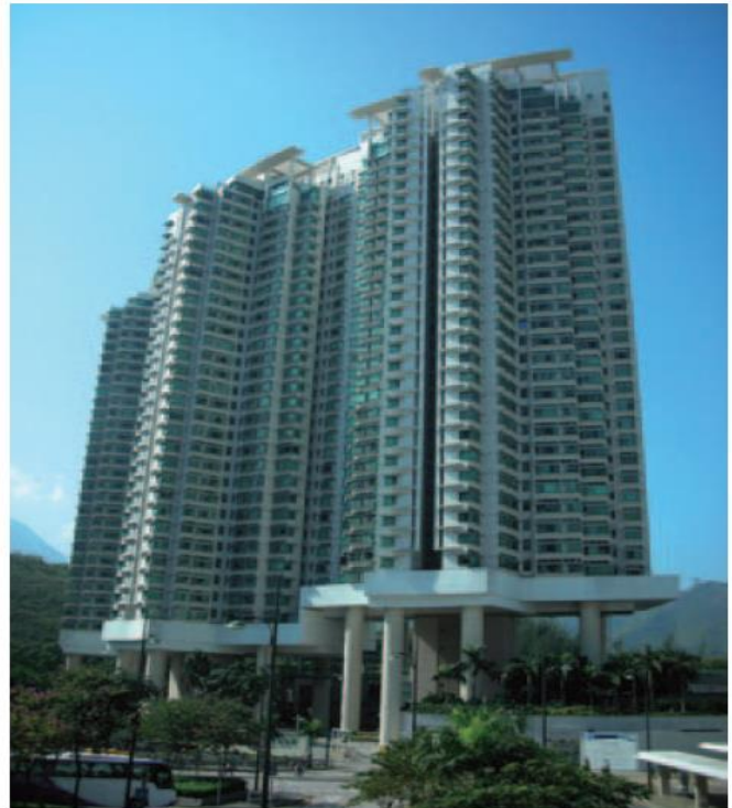
Figure 2.1. A residential building in Hong Kong having transfer structure at 1st floor level. (Su, R. K. L., & Cheng, M. H. (2009))
