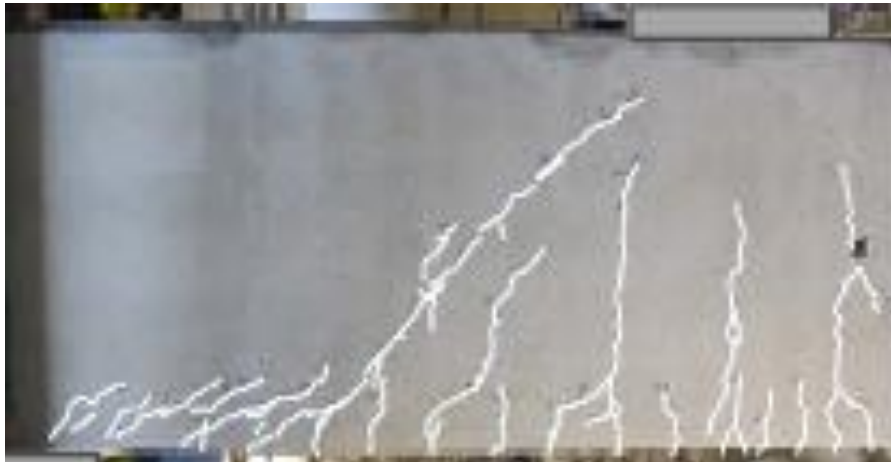
Figure 2.6. Developments of cracks in deep concrete specimen (David et al., 2008)
