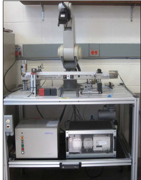
Fig. 2. Robotic arm is shown, controlling a conveyor line, with optical, proximity, and capacitive sensors. A Mitsubishi PLC is located on a shelf below the arm and to the right, and a Mitsubishi RV-M1 robotic unit is on the same shelf, to the left.
