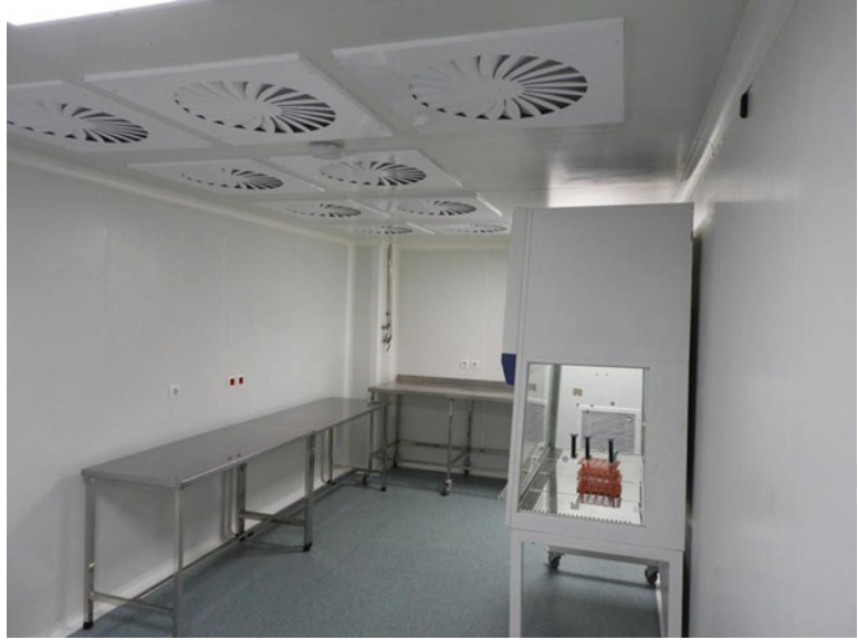
Fig. 1 Clean room as a GMP-compliant facility with controlled temperature, humidity, air pressure, and air particles can reduce contaminations in the manufacturing biomedical products process
