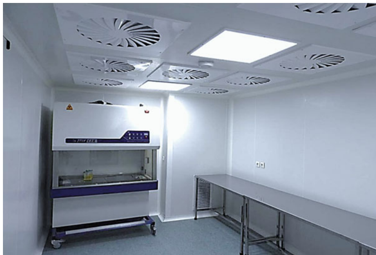
Fig. 1 Clean room (GMP) facility. Clean room is environmentally controlled aria which is required for manufacturing of biomedical products in accordance with GMP principles
