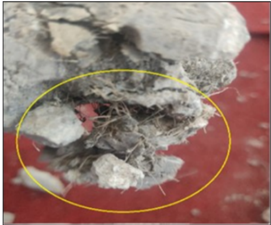
Hanging of small broken particles
