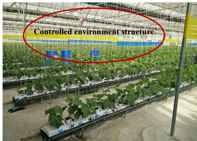
Figure 1.1: Hydroponic greenhouse structure
