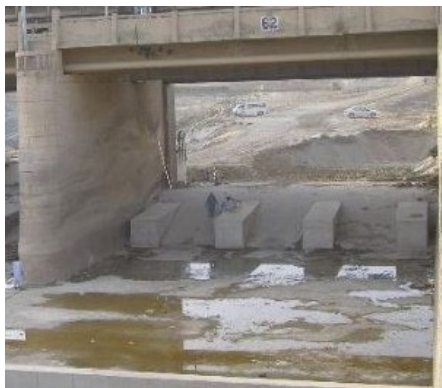
FIGURE 3.6: Existing appurtenances of barrage [43]
