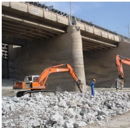
FIGURE 3.5: Dismantling of Baffle blocks [43]
