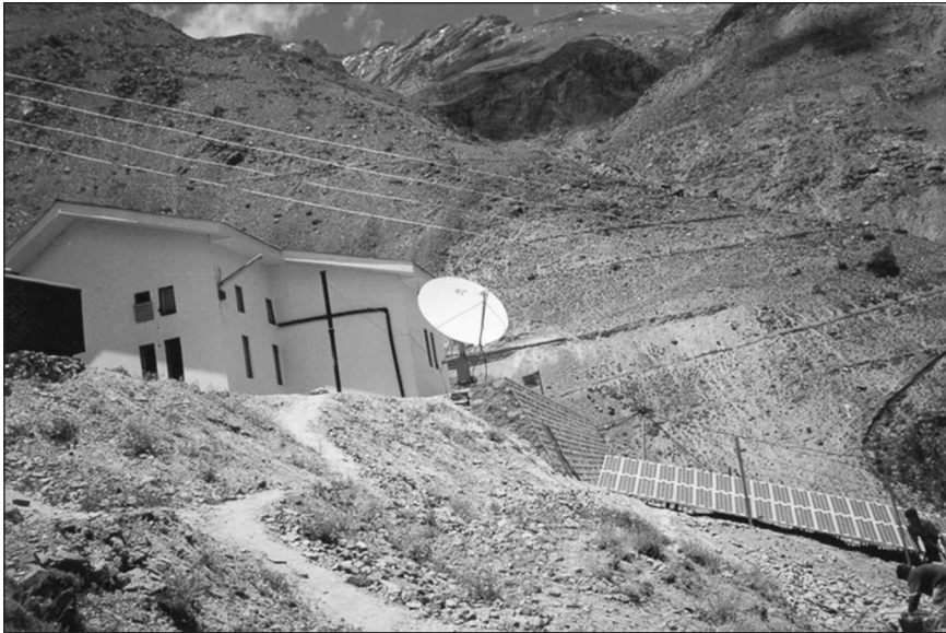
Figure 6.57 SPV for satellite earth station
