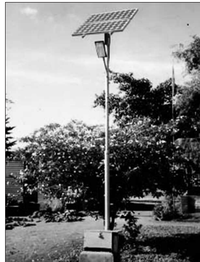
Figure 6.54 Pole mounted SPV lighting
