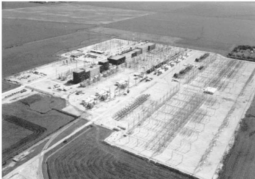
FIGURE 5.26 Dorsey Terminal of the Nelson River HVDC transmission system. (Photo courtesy Manitoba Hydro.)
