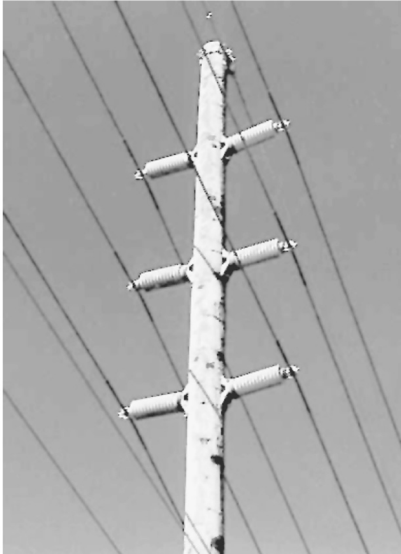
FIGURE 4.22 69-kV transmission line with post insulators.
