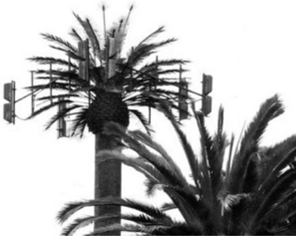
Figure 1-6 A ubiquitous cell phone tower, disguised as a palm tree. The one in the foreground is real. Photo by Daly Road Graphics.
