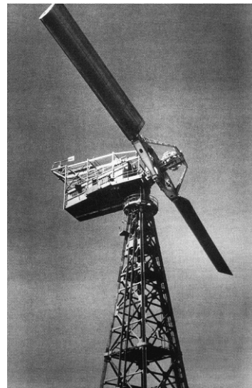
d) Smith-Putnam wind turbine (1,250 kW, D = 53 m, USA 1941)
