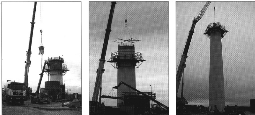
Fig. 3-54 Tower made of in-situ concrete with jacking formwork (Pfleiderer)
