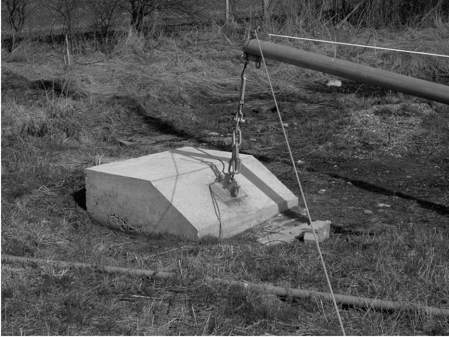
Fig. 3-60 Foundation for guyed tubular steel pole
