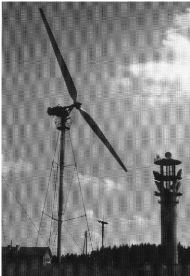
c) Hütter wind turbine (100 kW, D = 34 m, D 1958)
