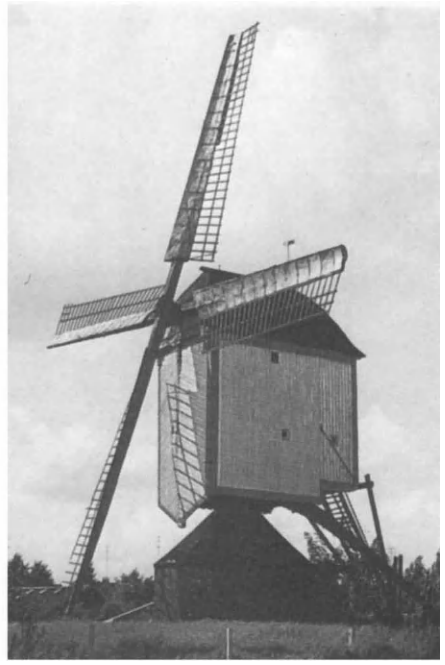
2. Rotating-caged windmill.
