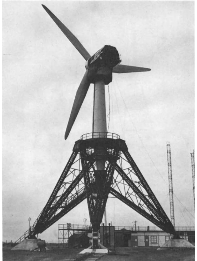
11. Best-Romani wind generator, 800 kW (France).
