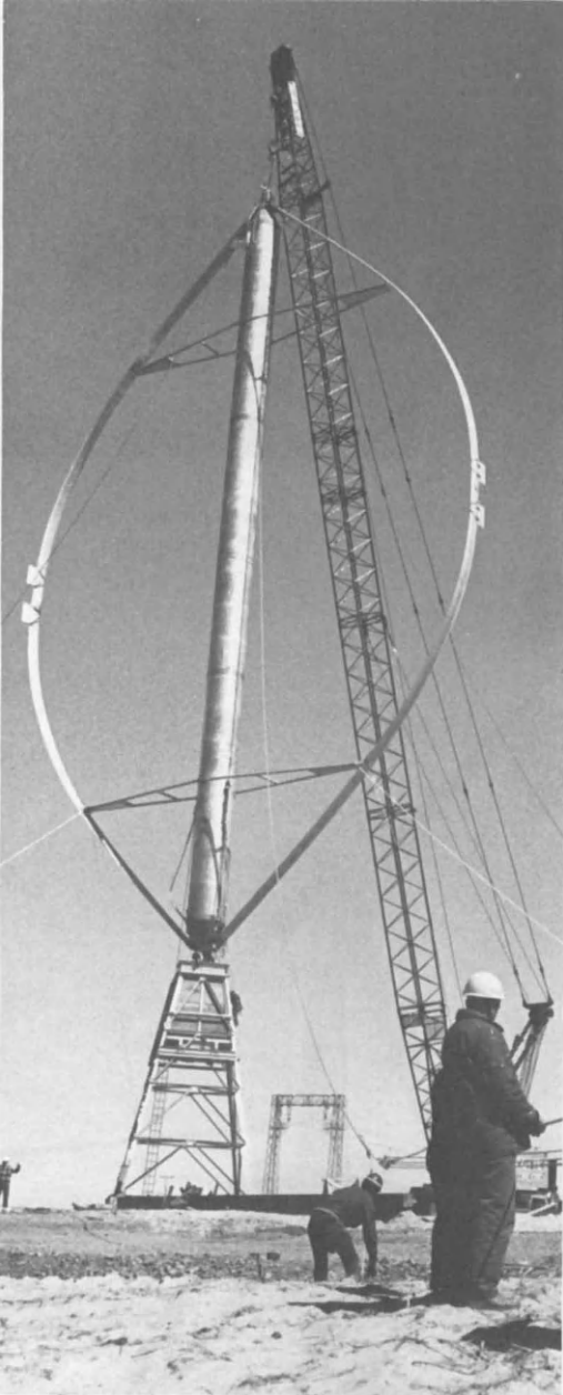
12. Darrieus rotor erected on the iles de la Madeleine, 200 kW (Canada).
