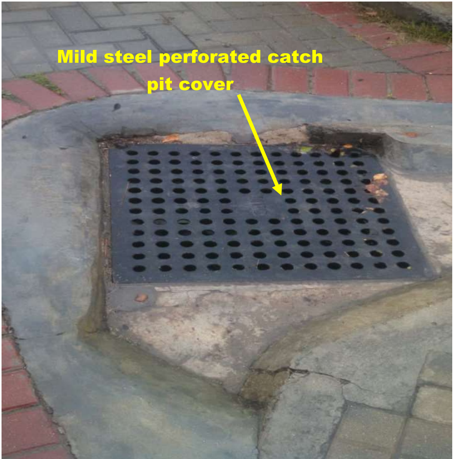
Fig P4: Close Photograph of mild steel perforated mild steel catchpit cover
