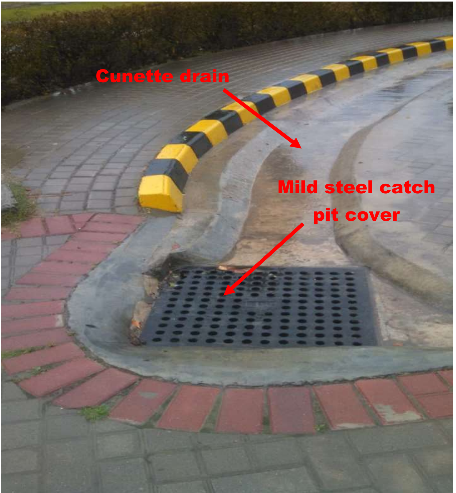
Fig P3: Photograph of Trapezoidal shape drain and perforated mild steel catchpit cover
